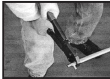
Grasp crimp ring with tool head and squeeze handles together until fully closed.
